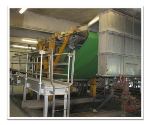
Digested solids are dewatered using existing belt filter presses
