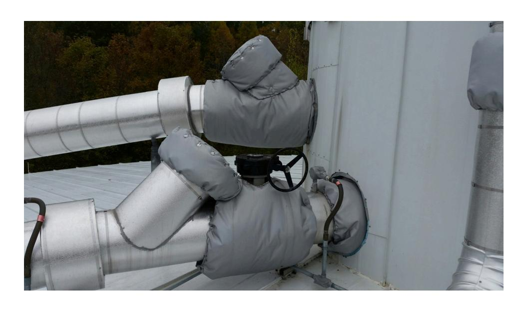
Normal Digestate Draw Off Point and Digestate Overflow
