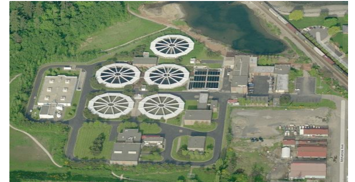
Post Point Wastewater Treatment Plant, Bellingham WA
