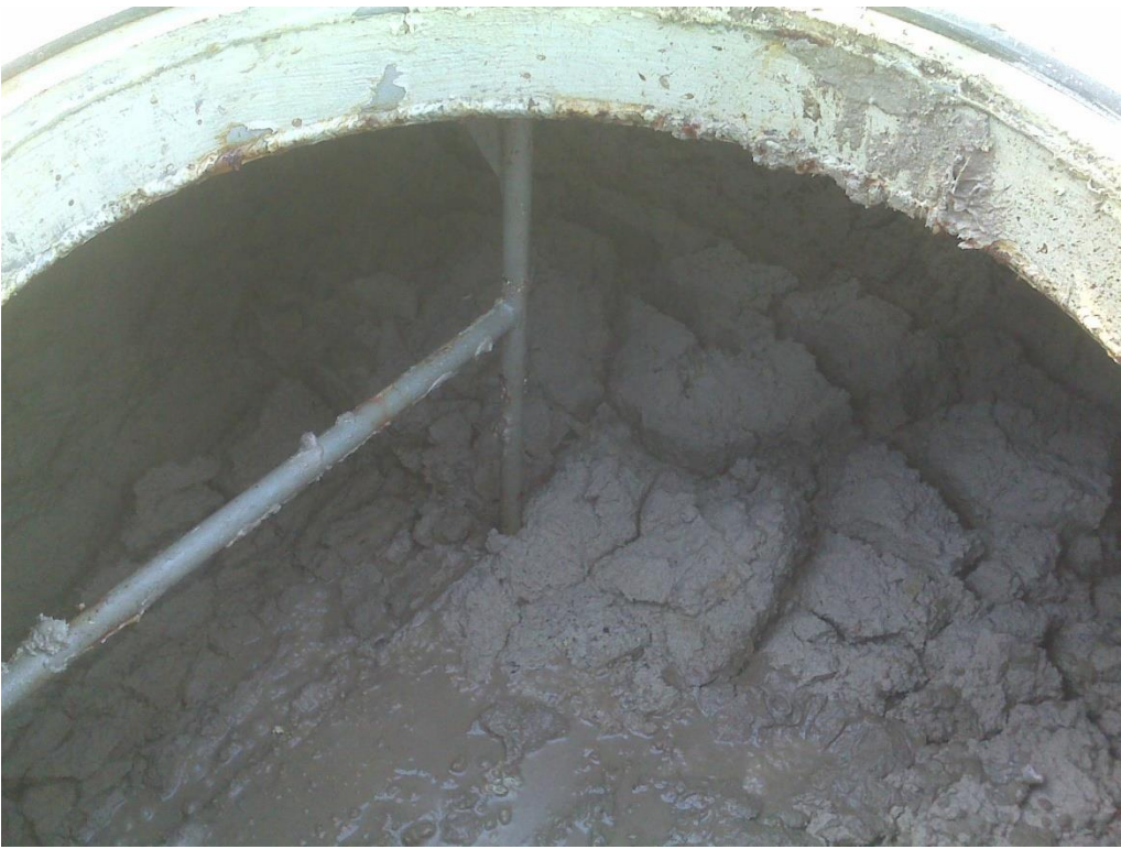
FOG floats when not adequately mixed
