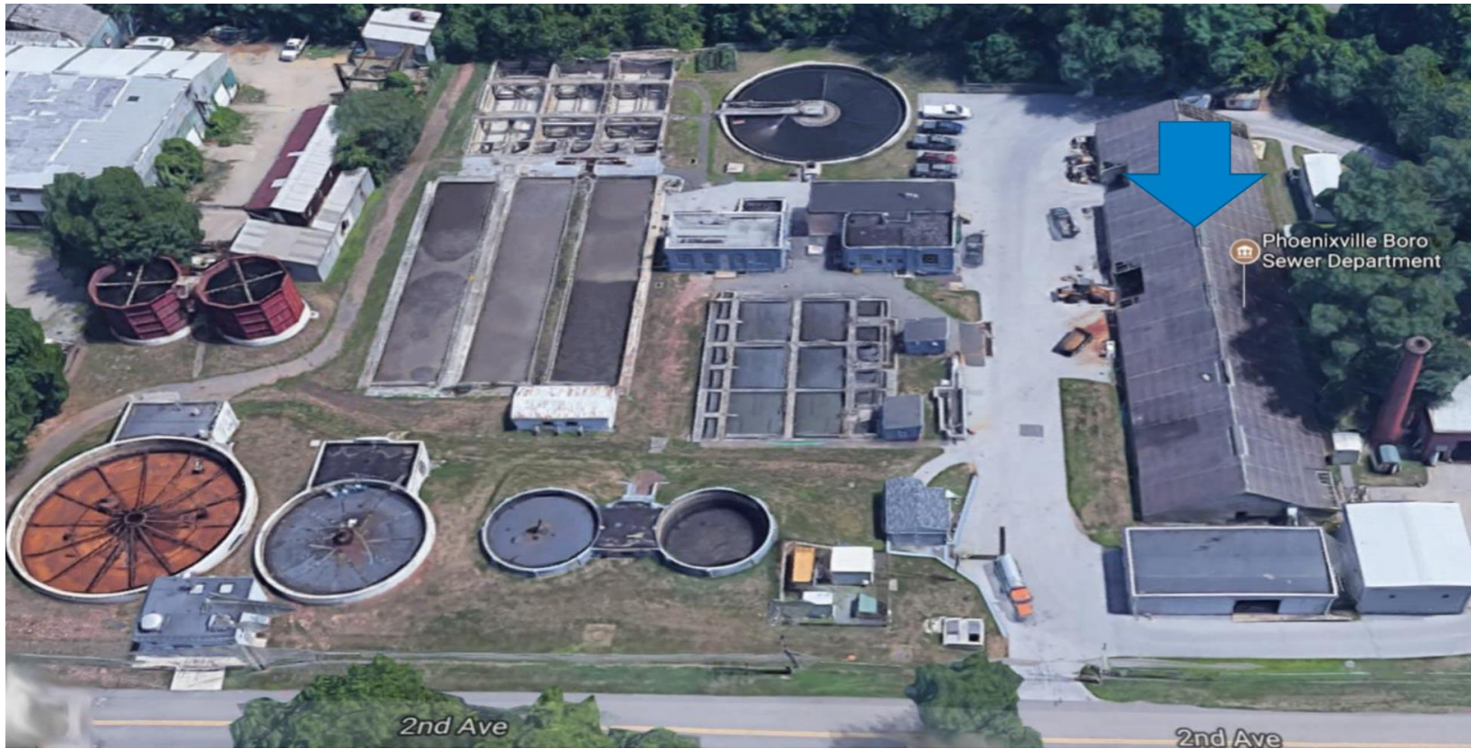
Borough of Phoenixville WWTP
