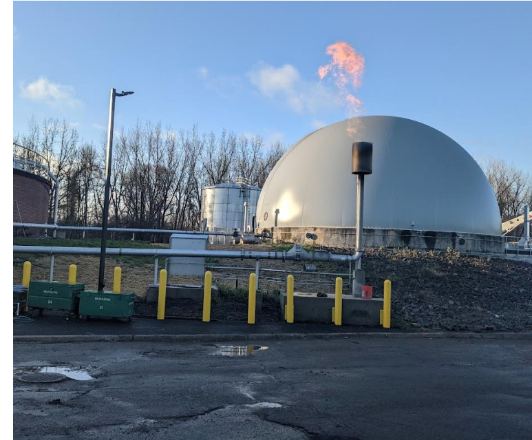
Biogas Storage in dual membrane cover
