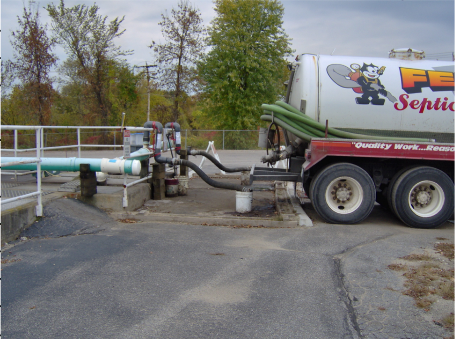
Delivering septage to a WRRF
